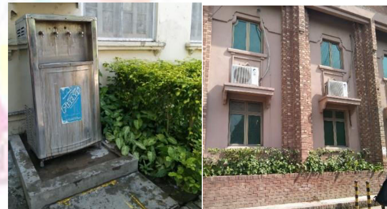
Water reuse from water coolers and AC unit
