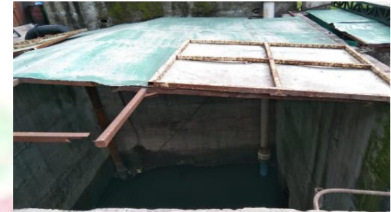
Septic tank for partial sedimentation of collected wastewater
