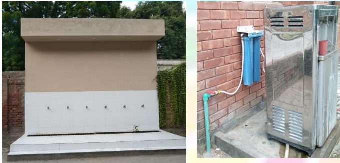
Water filtration plant and water coolers
